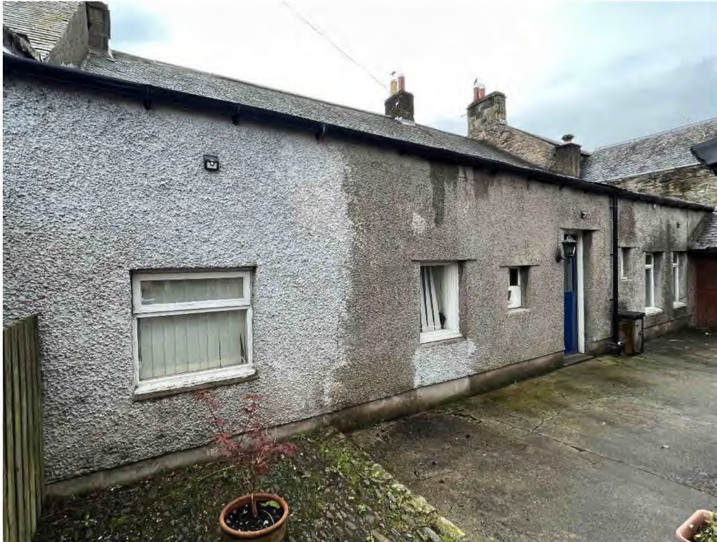
Figure 1: Rear of property
